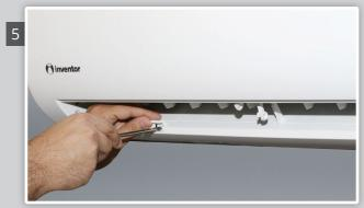
Remove the screw placed under the left cap.
