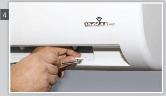
Remove the screw placed under the right cap.
